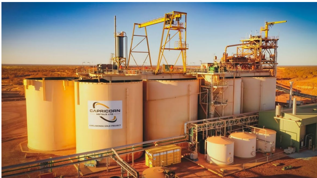
Additional CIL Construction at Karlawinda
